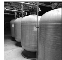
Cooling Tower Water Softener
